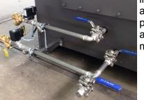
in the pipe line. The capacities of these flow regulators are fixed when the boiler is delivered. The discharge percentage will always be the same fixed value. Optionally, a heat exchanger can be supplied with which the make-up water is pre-heated by the drain water.
